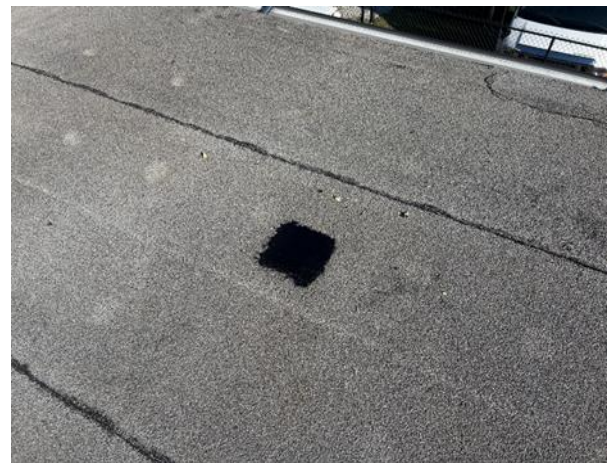
View of repair made at Core cut. Typical of both cores
