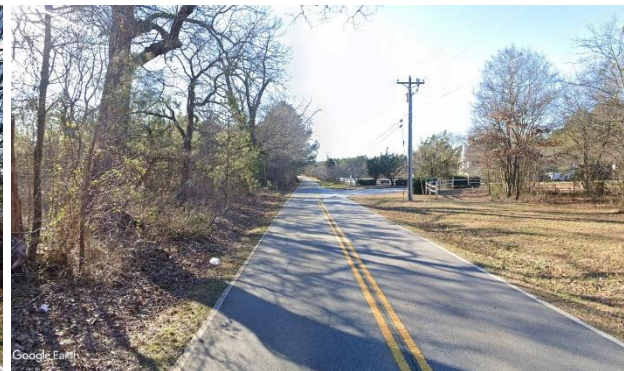
Old Covington Rd NE westbound approaching Horseshoe Springs Dr NE
