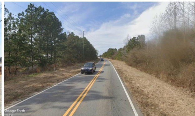
Old Covington Hwy SE westbound approaching Courtesy Pkwy SE
