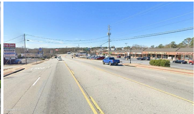
West Ave SW westbound approaching GA 20
