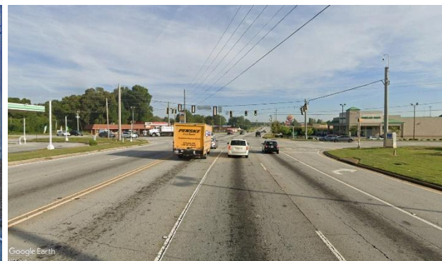
Salem Rd SE northbound approaching Flat Shoals Rd SE
