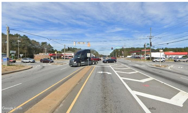
GA 20 northbound approaching Honey Creek Rd SE
