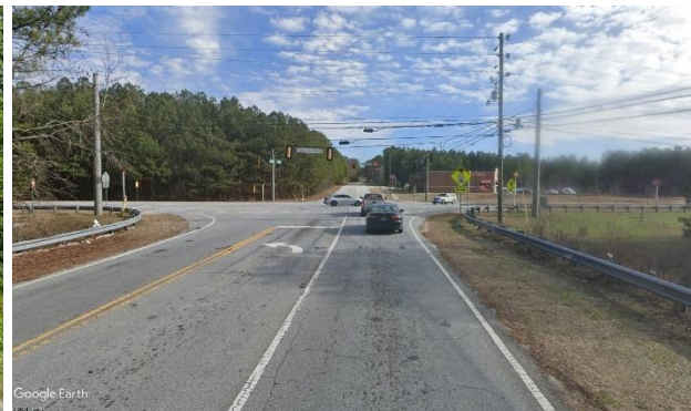
Hi Roc Rd NE eastbound approaching GA 138
