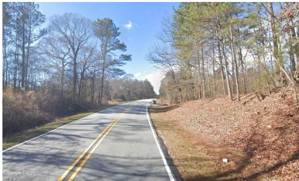
E Fairview Rd SW westbound approaching Union Church Rd SW
