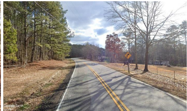
E Fairview Rd SW eastbound approaching Woodside Dr
